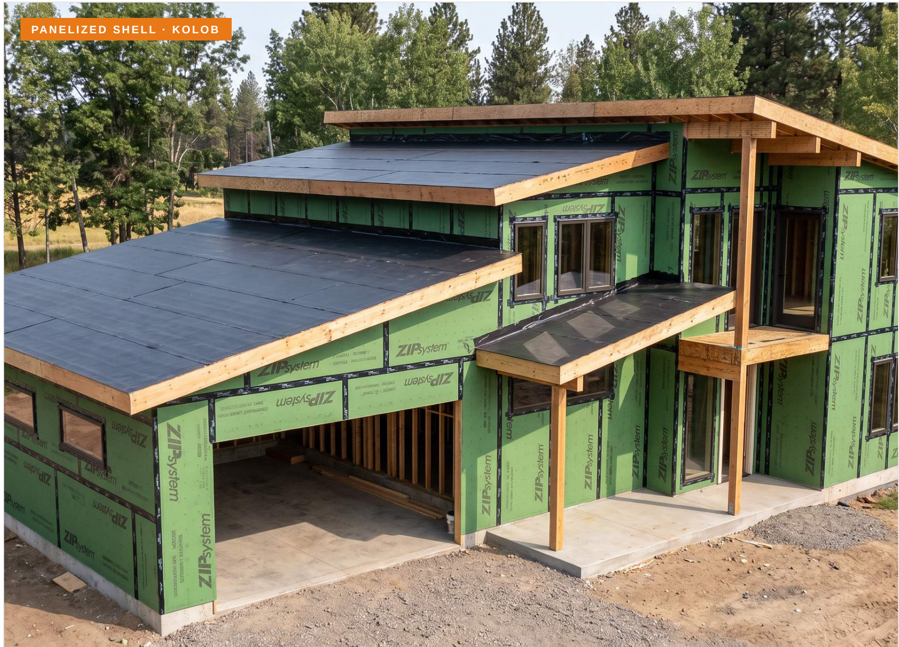
Kolob panelized shell on site — both stories standing, ZIP System sheathing taped, stepped shed roofs with underlayment down, the covered entry roof on a timber post, the balcony platform framed, and the 2-car garage bay open. Windows and doors shown are an optional add-on and are not part of the base kit.
